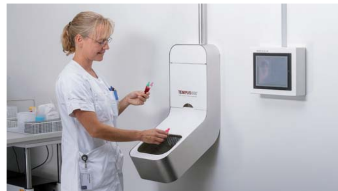
Samples arrive in the Receiving Tray where they are retrieved.
